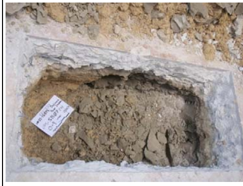
Photo 14. SB07 Hand dug service pit to 0.9m bgl
